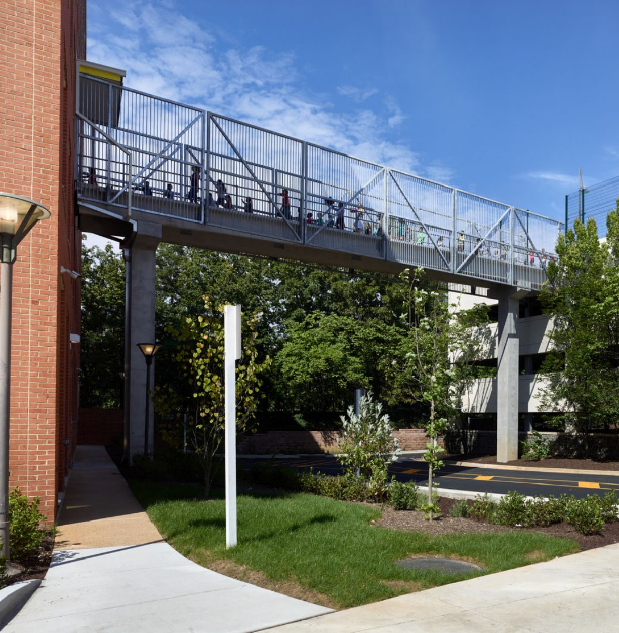
Connecting Bridge & Gym Addition
